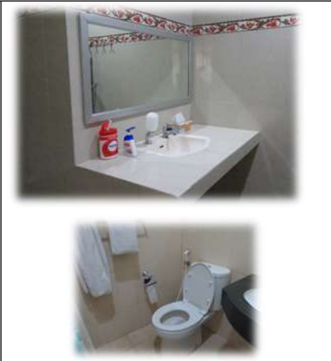
Figure 02: Water efficient appliances have also been used in authomatic stopped water tap in wastafel and Toilet flush
