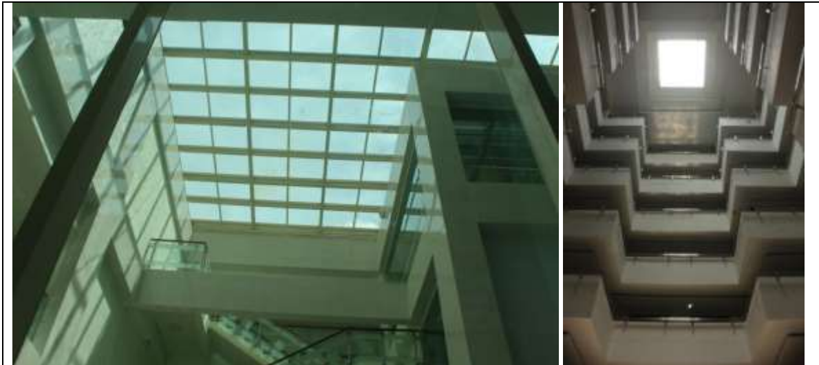
Figure 3. The use of glass material for the wall and roof as a Natural lighting is applied to the Library Building, Medical Faculty Building, the Post Graduate Building, and others.
