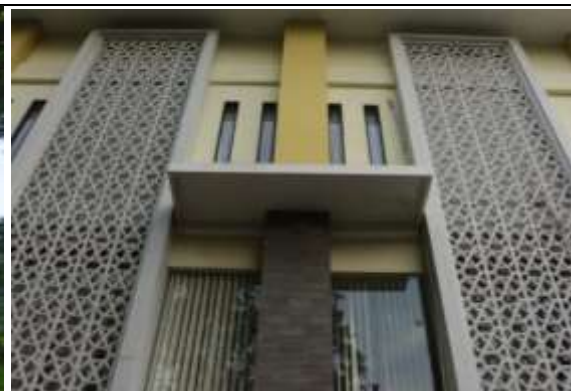
Figure 1. Natural ventilation by the use of roster in the UNS Inn
