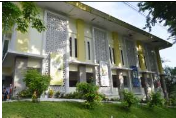
Figure 1. Natural ventilation by the use of roster in the UNS Inn
