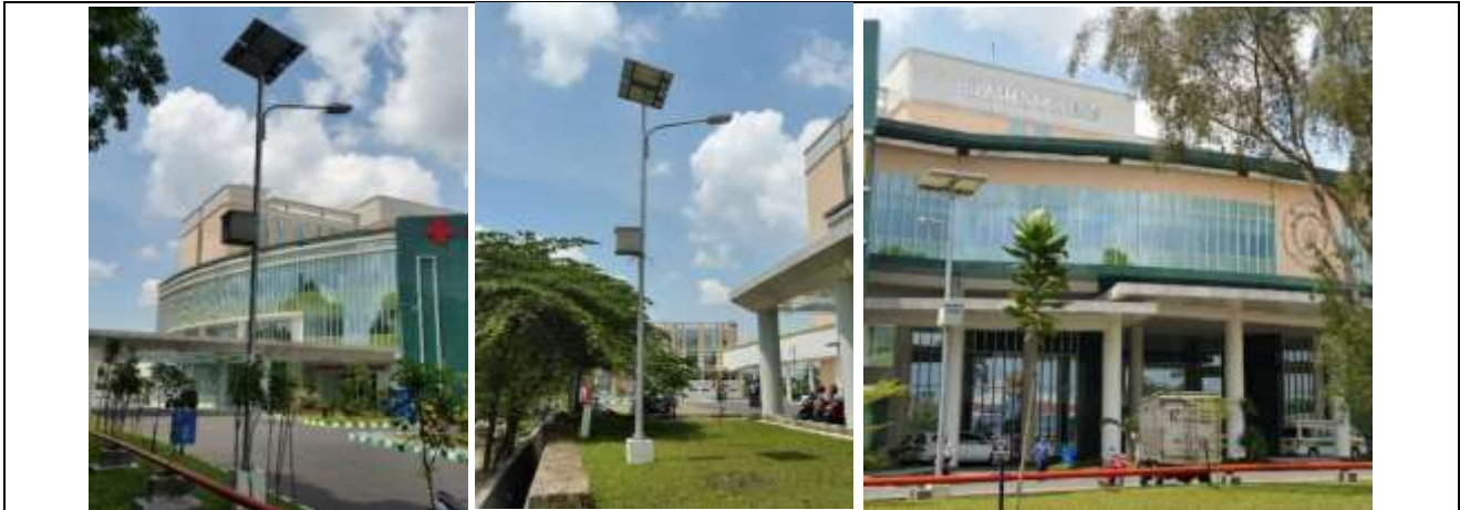
The Solar power energy is also applied as outdoor street lighting in the UNS University Hospital.
