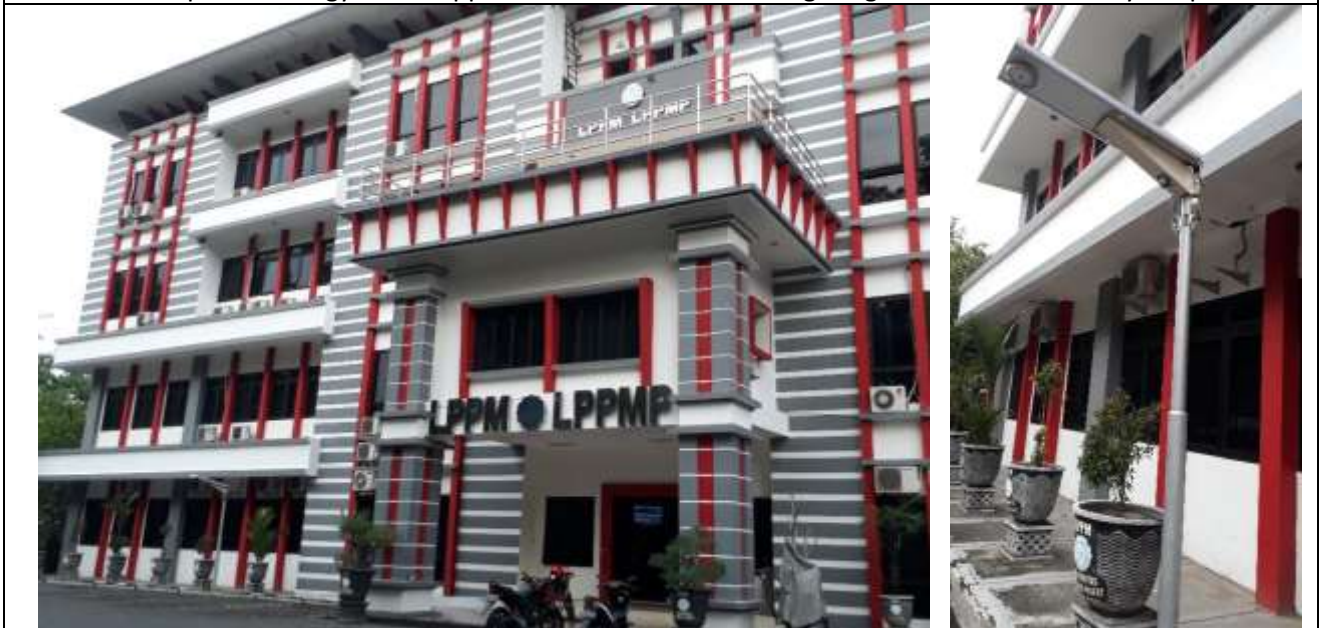
The Solar panel for the street lighting is applied in the Research and Development Services Building (LPPM) UNS Surakarta.
