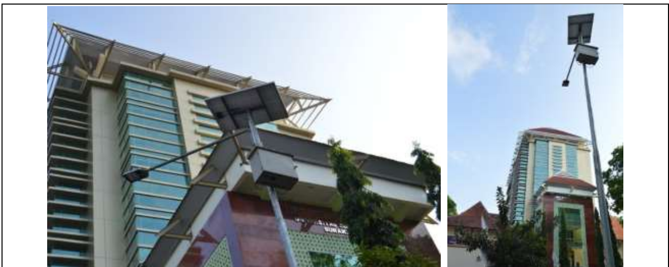
The Solar power energy for outdoor street lighting is applied in the Library Building.
