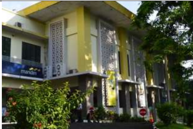
Figure 5. Smart Building implementation in the UNS Inn
