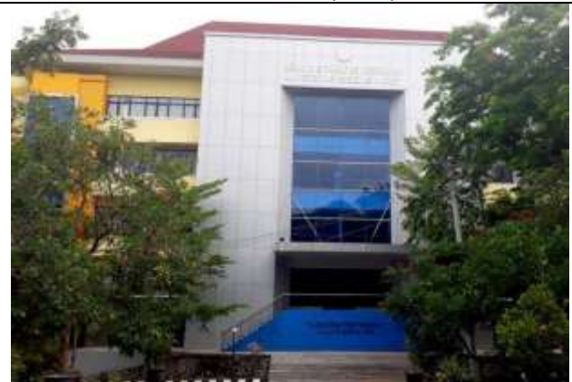
Figure 4. Smart Building implementation in the Building E, Faculty of Agriculture UNS
