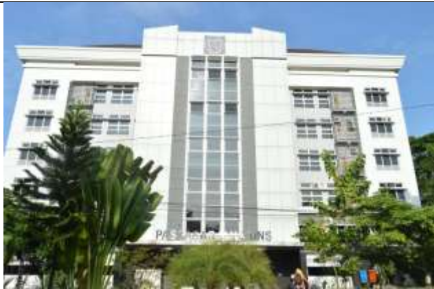
Figure 5. Smart Building implementation in the Post Graduate Building UNS
