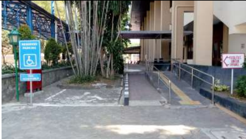
Figure 3. Pedestrian area is provided by ramps and guiding block for safety of people having physical disabilities
