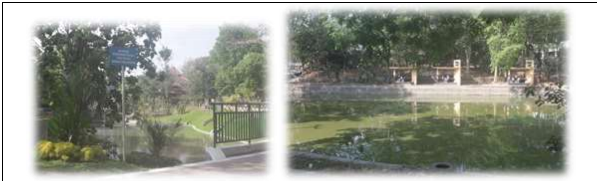
Figure 4.1. UNS has 2 ponds, which have function for water harvesting during rainy season. This also improves process of water infiltration.
