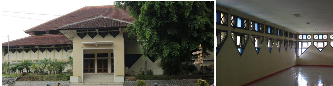
Figure 2. Natural Ventilation is also applied in Student Center Building by using permanent windows, which flow natural air circulation.
