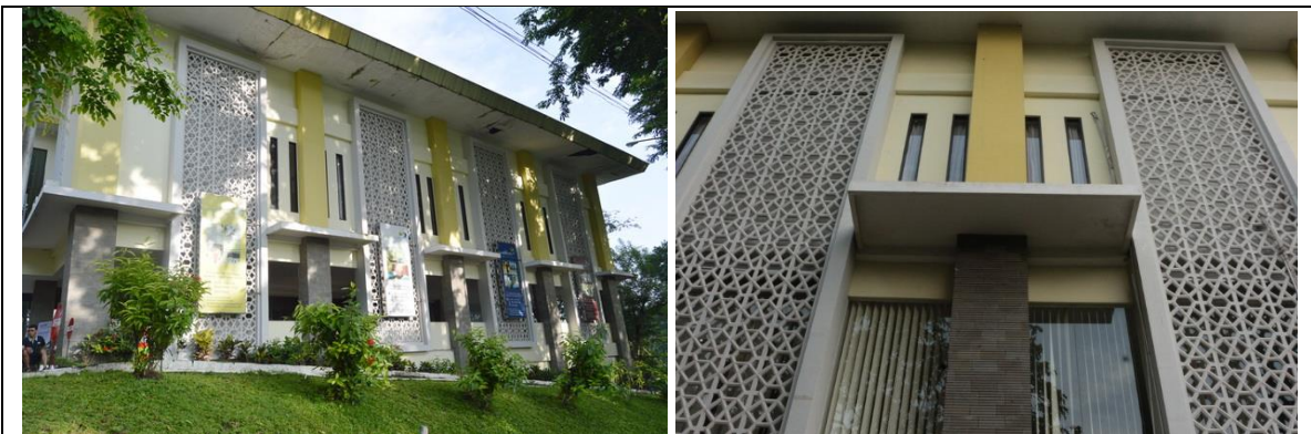
Figure 1. Natural ventilation is applied in UNS Inn by using Roster Bricks.
