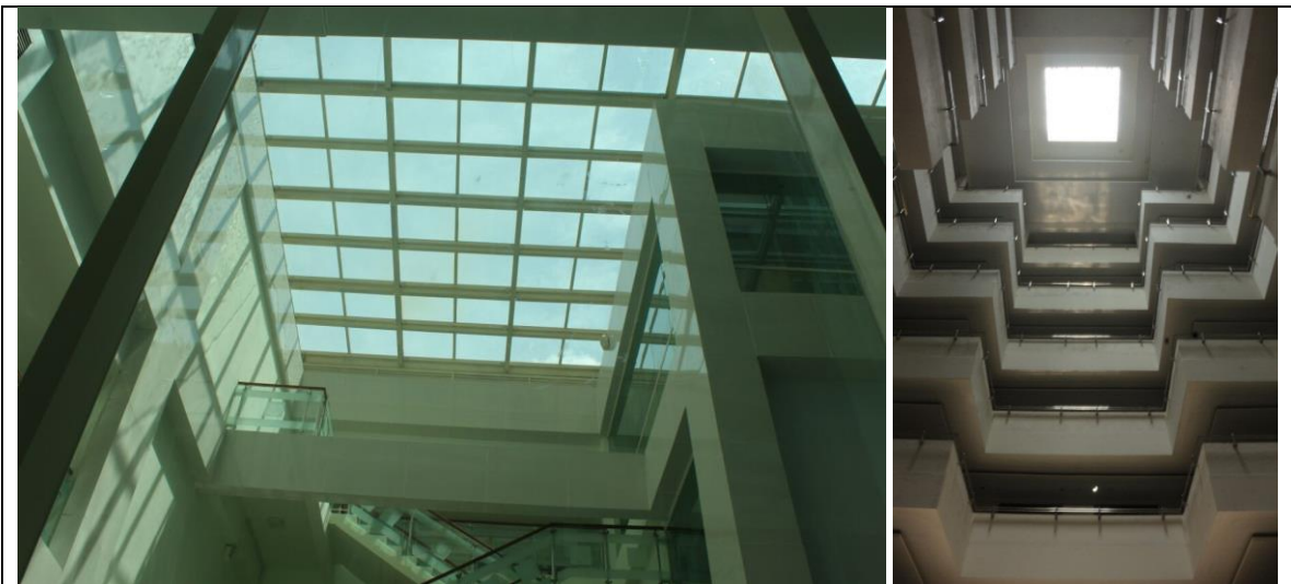
Figure 3. Natural lighting has been applied by using glass natural light reflector for roof and wall in Library Building, Faculty of Medicine, Post Graduate Building and other buildings.
