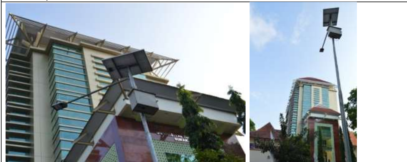
Figure 02. Solar System has also been used for Street Lighting in front of Library Building.
