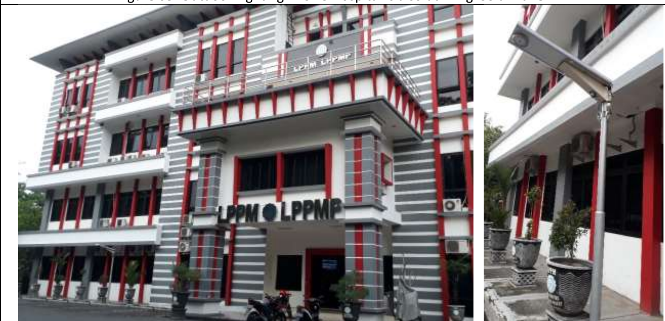
Figure 04. Solar panel is also applied for outdoor lighting in LPPM UNS Building .
