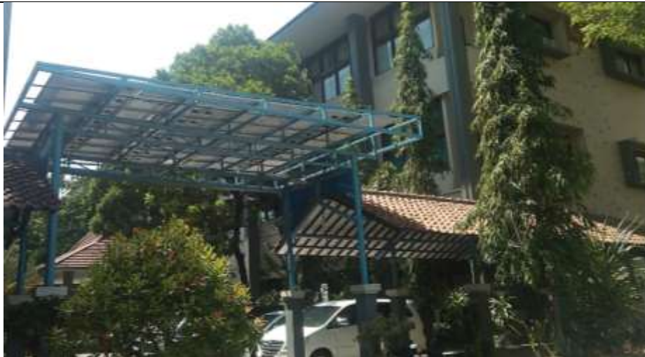
Figure 05. Solar panel is used in Faculty of Engineering UNS.
