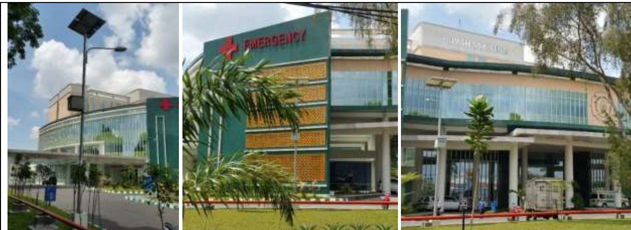
Figure 03. Outdoor Lighting in UNS Hospital is also utilizing Solar Panel .
