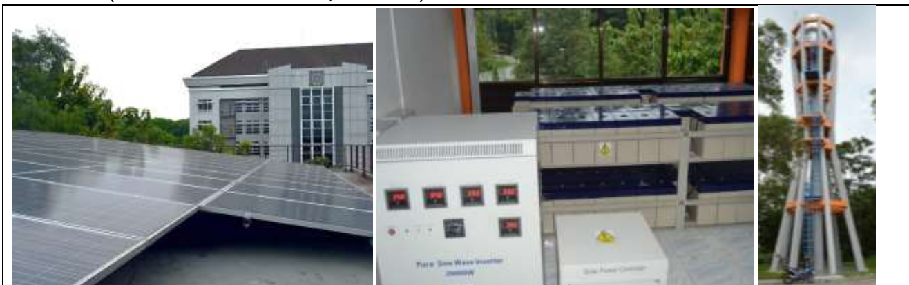
Figure 01. Solar Panel has been applied for Drinking Water Treatment System (SPAM : Sistem Pengolahan Air Minum)
