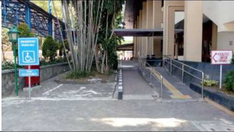
Figure 3. Pedestrian area is provided by ramps and guiding block for safety of people having physical disabilities
