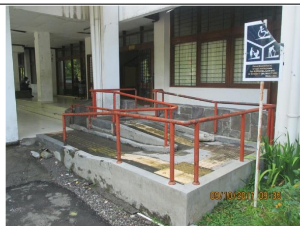
Figure 2. Universitas Sebelas Maret, Indonesia also provides Diffable Ramp for easy access from frontyard to the building for diffable people
