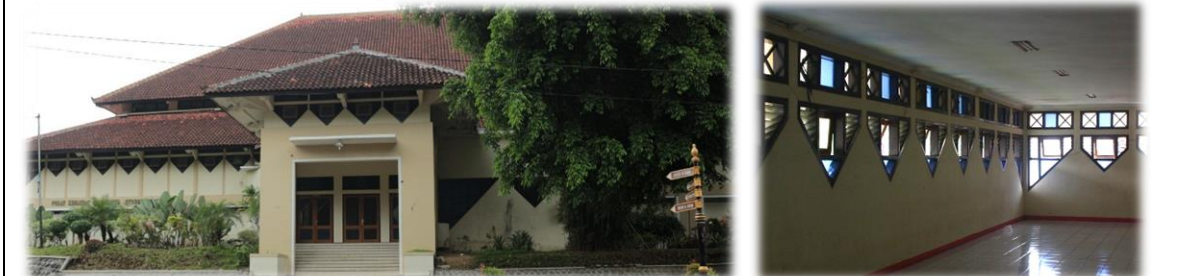
Figure 2. One of buildings in UNS, for example Student Center Building uses natural ventilation windows for having natural crossing ventilation daily. .
