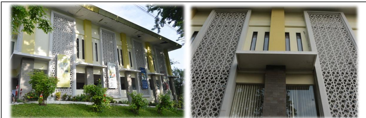
Figure 1. Some buildings in UNS uses roster as natural ventilation as applied in UNS-Inn
